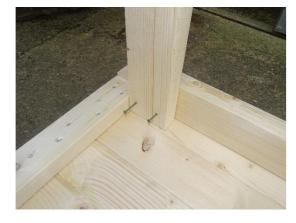
Ensure the leg is pushed into the corner and secure with the supplied screws.
