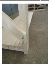
Ensure the brace is lined up with the front of the leg and secure into place with the screws supplied.
