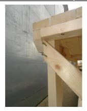
Ensure the brace is pushed into the top corner and screw into place.
